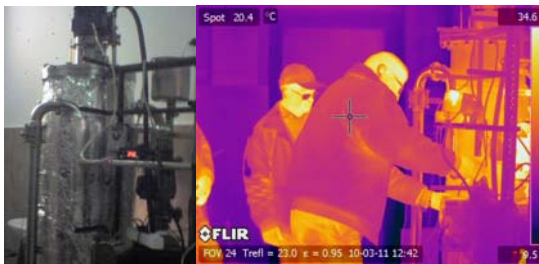
Fig.1. Accomplishment of heat insulation of the bioreactor to compensate the heat losses
